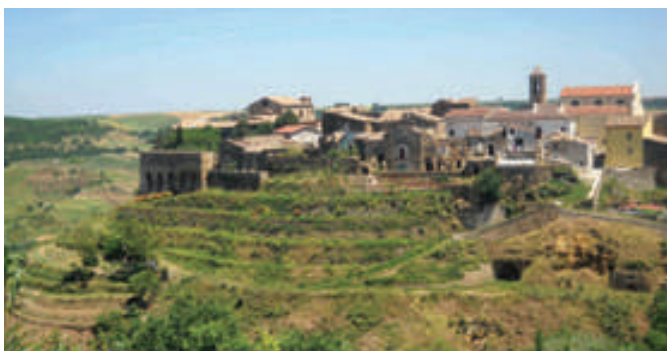
Special maintenance and stabilization of the cliff under the historical site in Genzano di Lucania (PZ).
