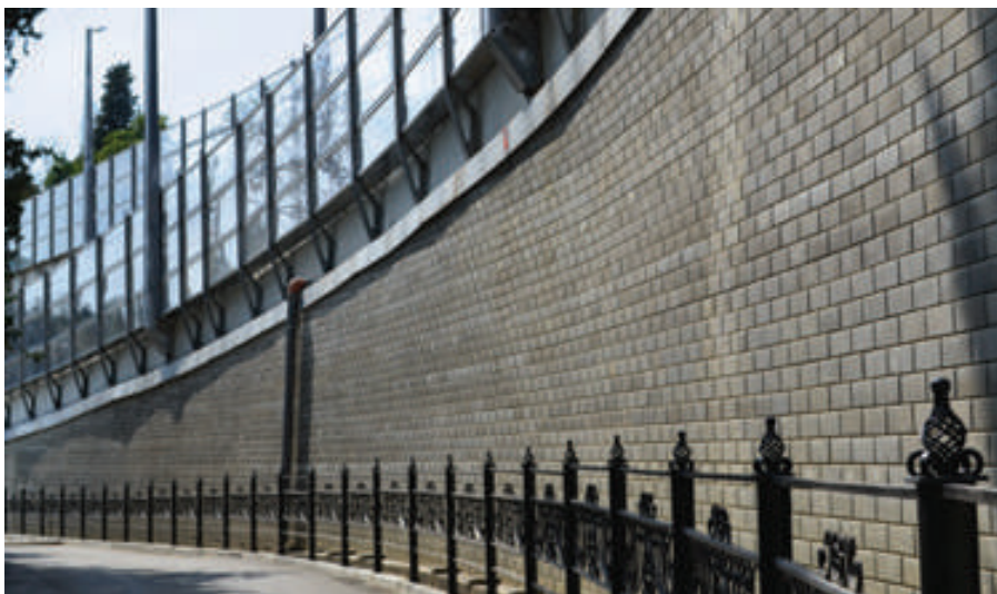
Sochi, Russia. Work carried out for the Olympics.
