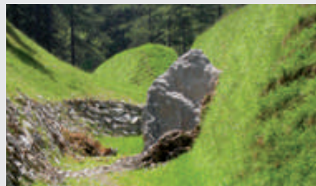
A rocky boulder stopped by TENAX reinforced rockfall barrier in the Créton area of Rhêmes Saint-Georges municipality (Italy).
