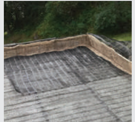
Placement of steel drainage tiles.
