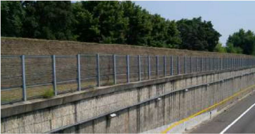
Works on the A51 ring road in Milan for the construction of a noise barrier using vegetated reinforced slopes, to protect adjacent residential areas. The structure is approximately 300 meters long and 3 meters high.
