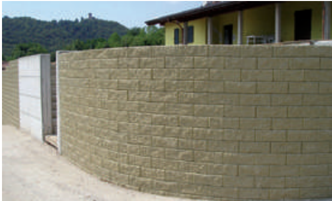
Construction of curved sections.
