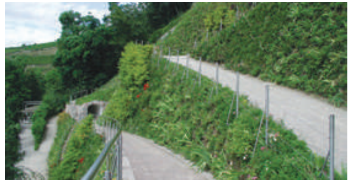
Terraced gardens using TENAX reinforced slopes at Merano Botanical Garden, Italy.
