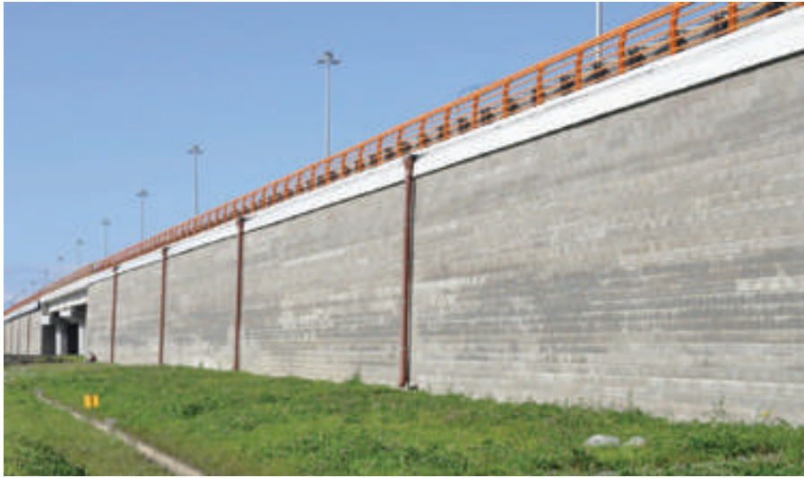
St. Petersburg ring road, Russia. Geogrid reinforced wing wall.
