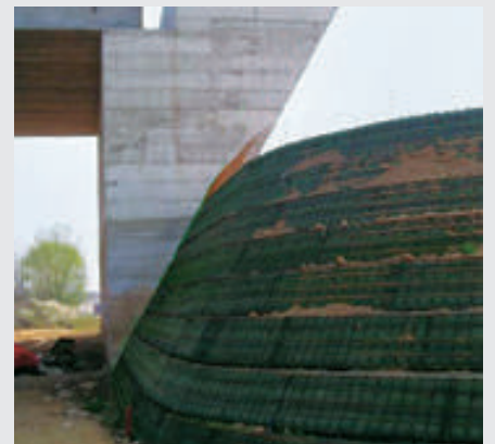
Detail of the connection between reinforced slope and existing concrete structure.
