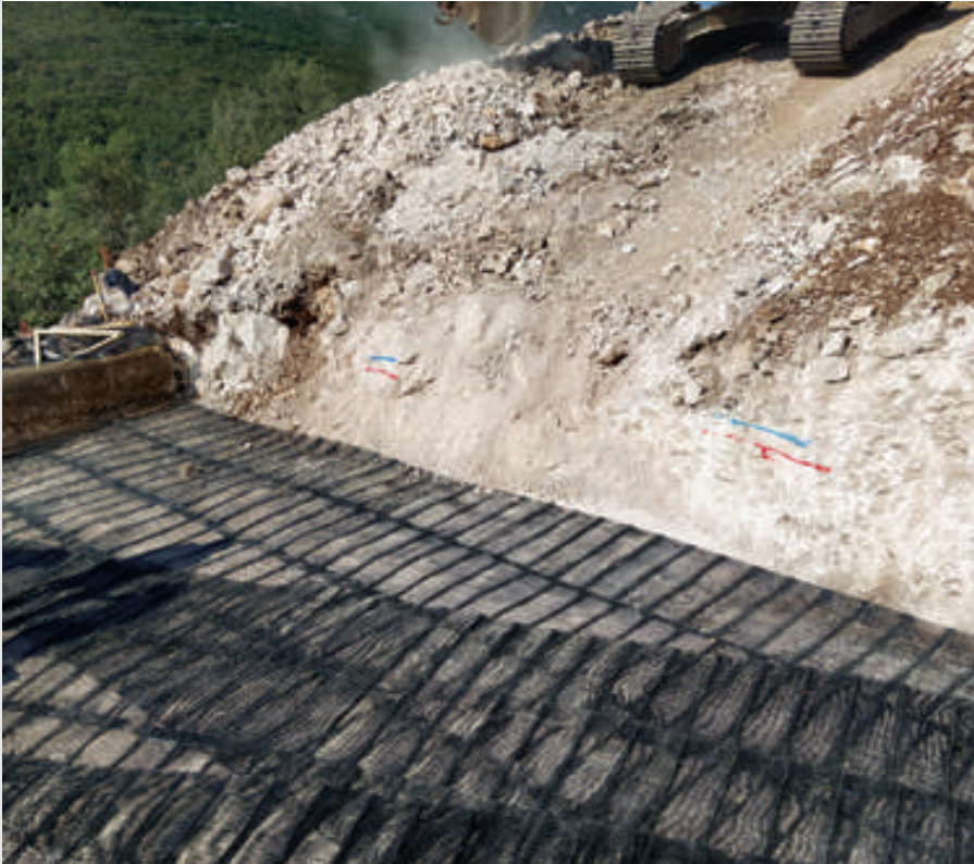
Geogrids are overlapped at the front or back depending whether the section is concave or convex.
