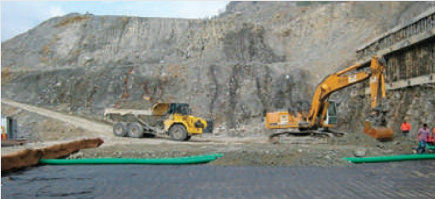
Placement of drainage pipes.
