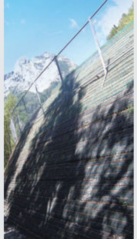
Safety-rules compliant railing on construction site.
