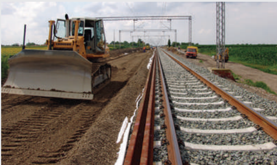
Vinkovci/Tovarnik, Croatia. Reinforcement of the railway embankment with TENAX geogrid. 185,000 m 2 of geogrid has been installed for the Croatian railway.
