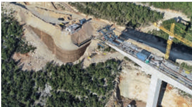
Bridge abutment, Peljesac Bridge, Croatia.
