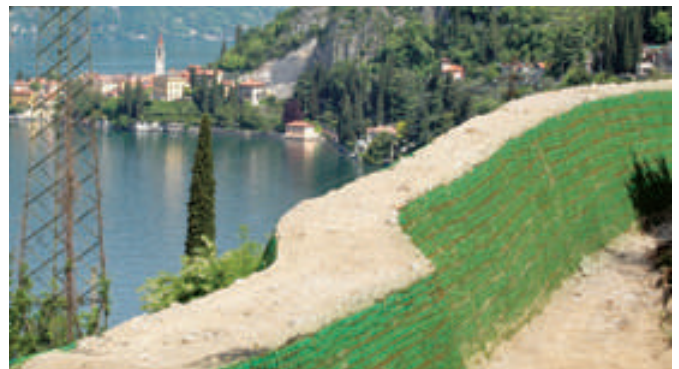
Rockfall barrier, Varena (LC).
