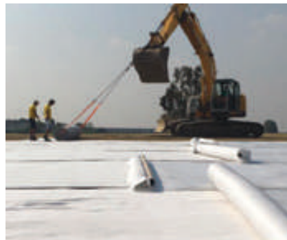
3 INSTALLATION OF THE GEOCOMPOSITE FOR DRAINAGE OF INFILTRATING RAINWATER
