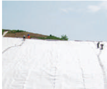
1 INSTALLATION OF THE GEOCOMPOSITE FOR BIOGAS DRAINAGE
