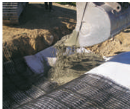
5 ANCHORAGE OF THE COMPLETE COVERING SYSTEM IN APPROPRIATE ANCHOR TRENCHES, IF NECESSARY, FILLED WITH CONCRETE
