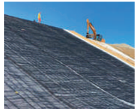
4 LAYING OF THE “GRIPPING” AND REINFORCED 3D GEOMAT
