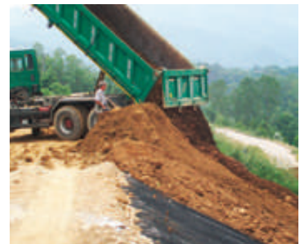
6 SPREADING OF THE UPPER LAYER OF VEGETATIVE SOIL COVER
